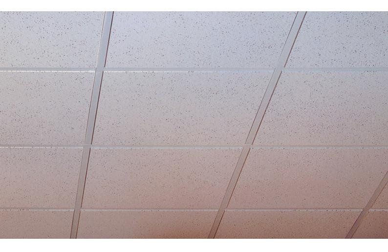
Taiga Perforated Acoustical Ceiling meets specifications in accordance with ASTM E1264 and EN13964.
